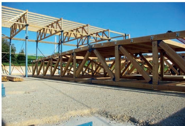
Demonstration construction site of an industrial building with a wooden framework (Douglas fir) in Castres (81), a project cofunded by Europe and promoted by the association Filière Bois Haut Languedoc Sud Massif Central association.
